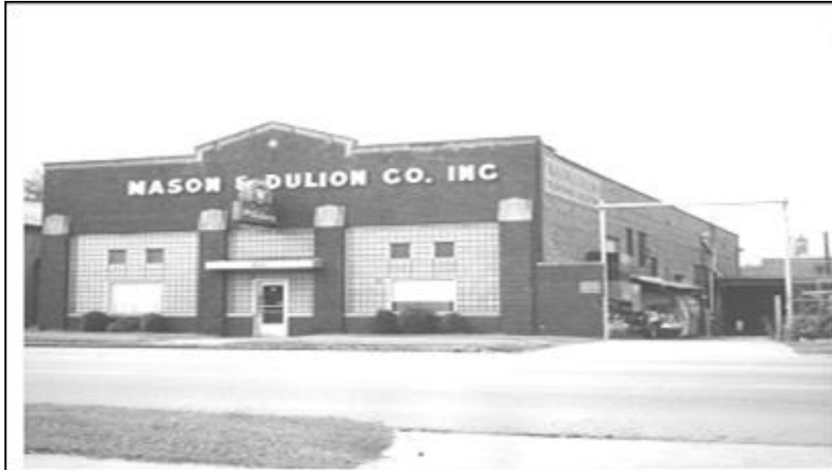
Mason & Dulion Co., Inc. building in Birmingham, AL.
